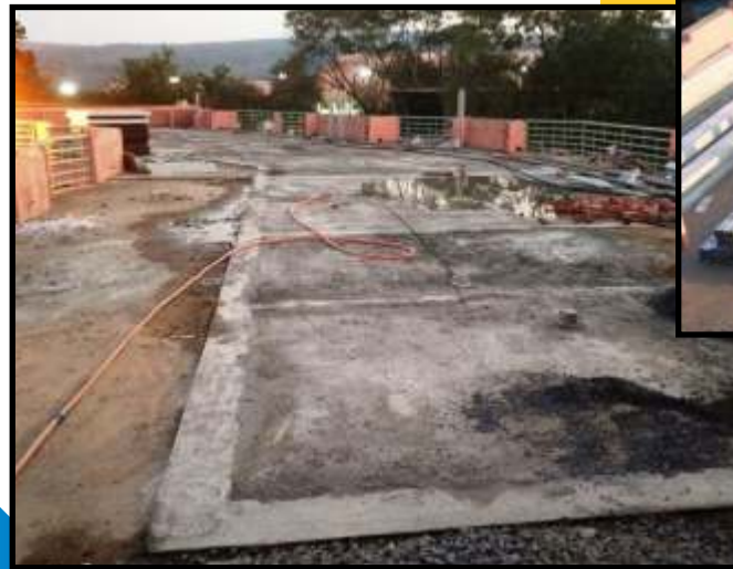
Water proofing & foundation 1
