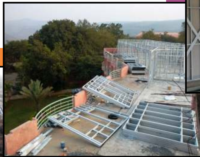
LGSF Erection 3
